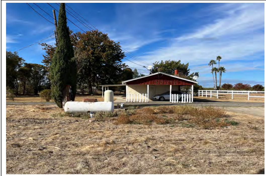
Building 1 looking east
