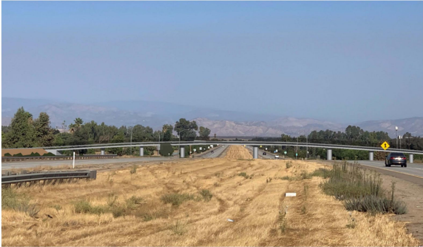
State Route (SR) 168 Enterprise Canal Pedestrian Bridge Project City of Clovis, CA Figure 2.2.1-3
