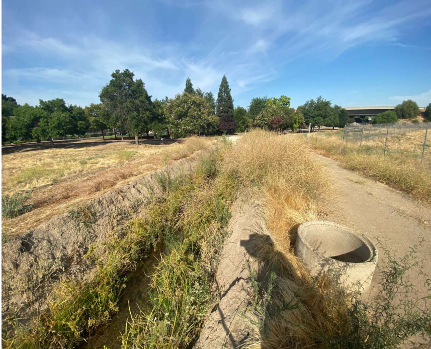
Photograph 3: Western segment of the ditch with valve on right, looking west.
