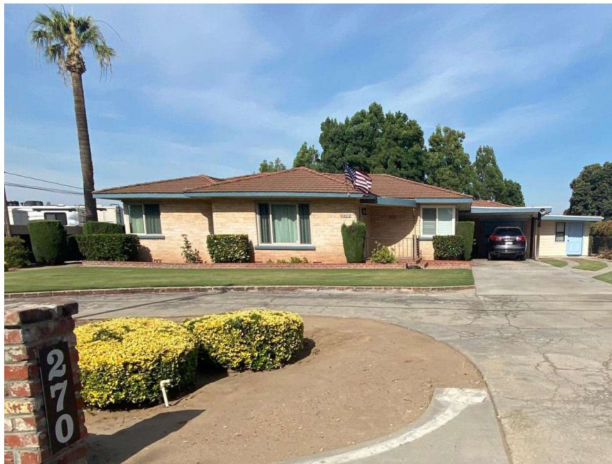
Figure 23: House located at 270 N. Clovis Ave. looking west.
