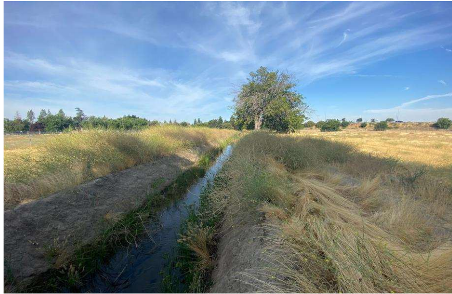
Figure 21: Central segment of the West Branch Clovis Ditch looking west.
