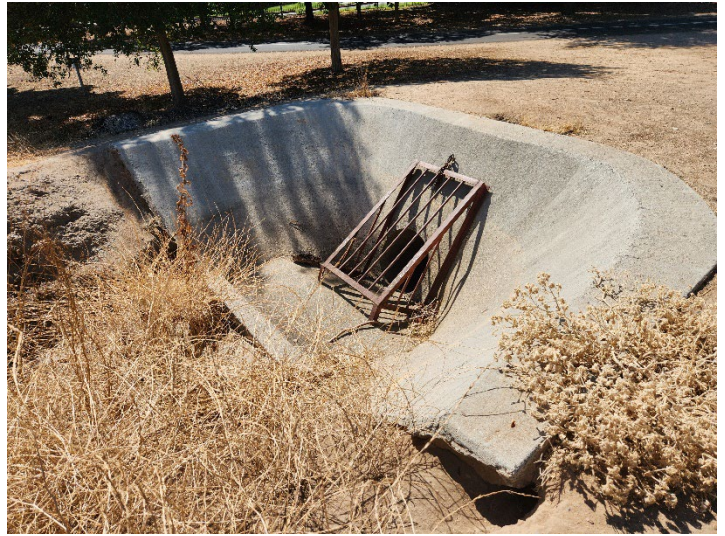
Outflow of West Branch Clovis Ditch.
