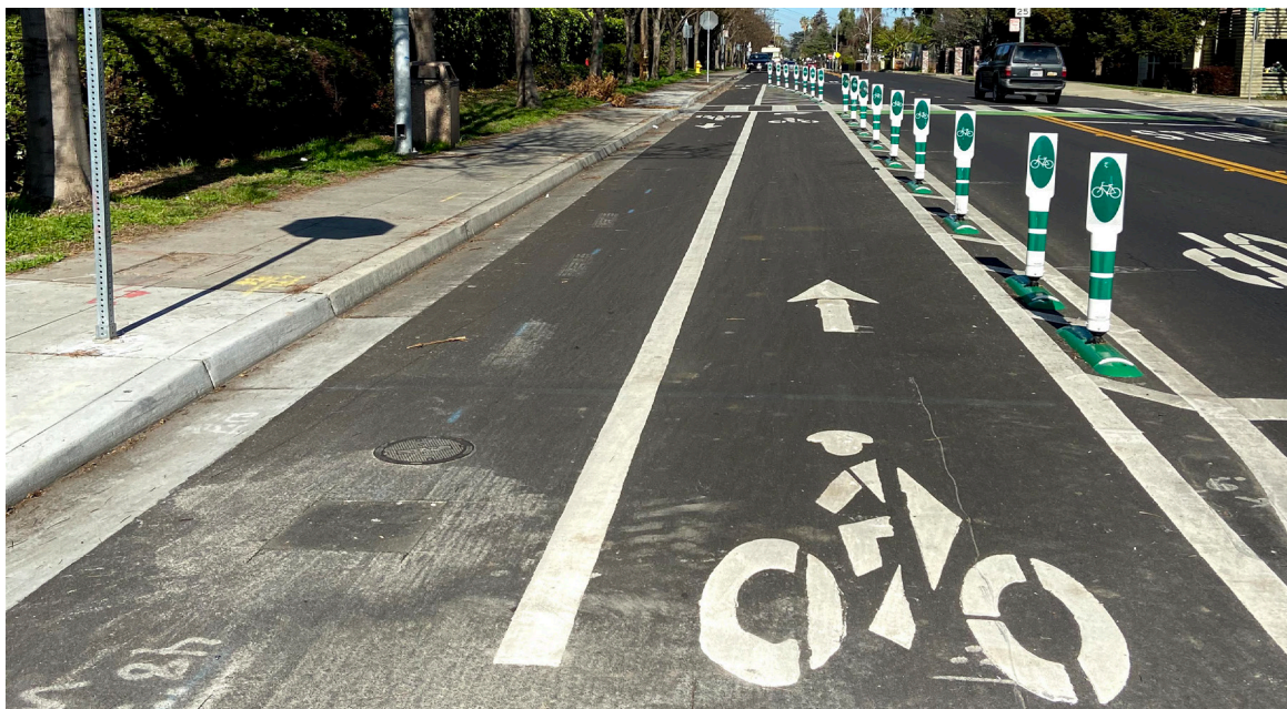
Figure 39: Two way separated bike lanes
