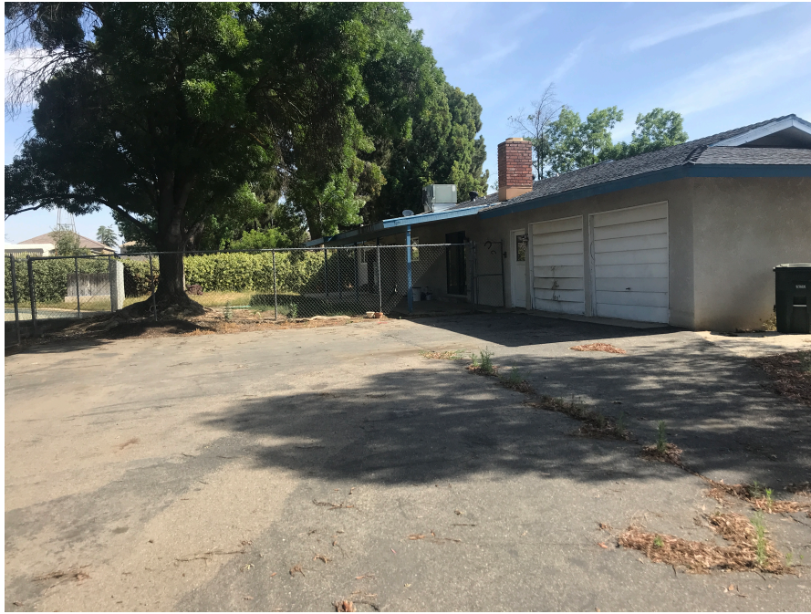
View of the developed area and ornamental landscaping associated with the development, facing north. May 5, 2022
