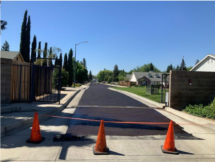
Slurry Seal Work June 2022
