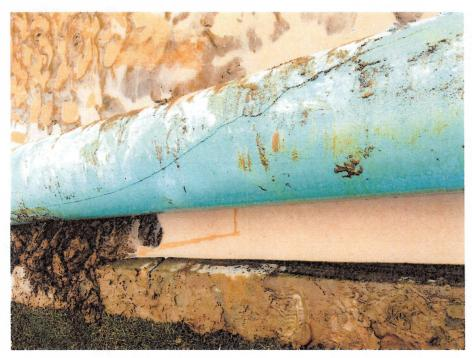
The damaged section of pipe was removed and a new section installed. The hole was then backfilled and compacted. Water service was restored to the area later that morning, and the #1 southbound lane of the road opened to traffic that evening.
